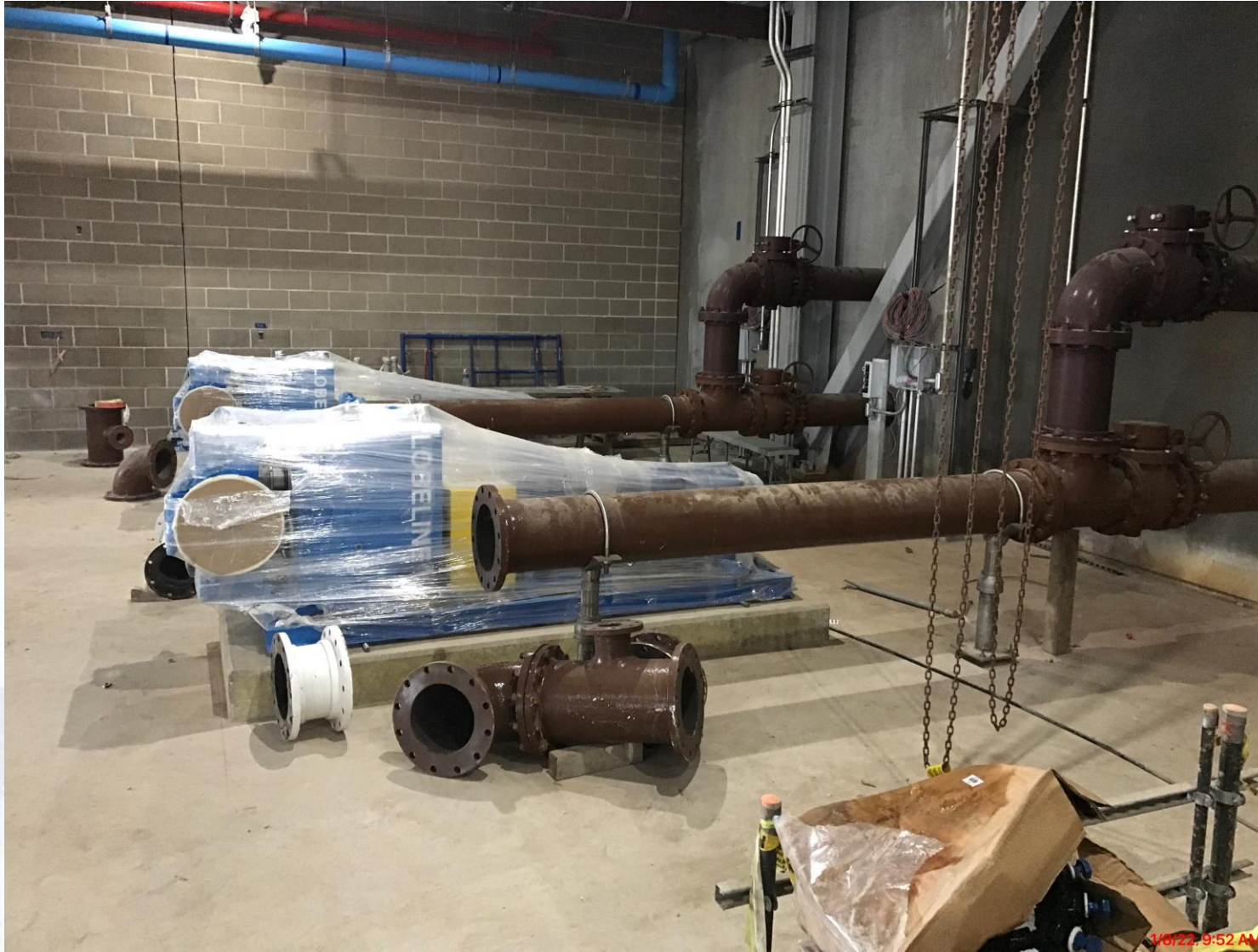
Delivery and installation of Swaby centrifuge feed pumps at Fac 520.
