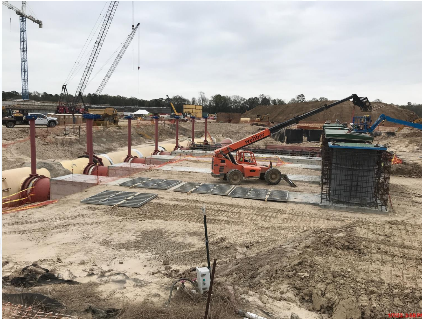
Continued backfilling at Fac 402.
