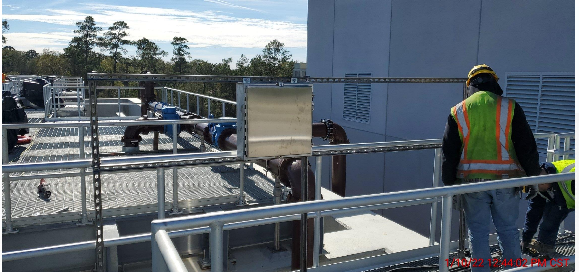
Continued process pipe installation at Fac 510.
