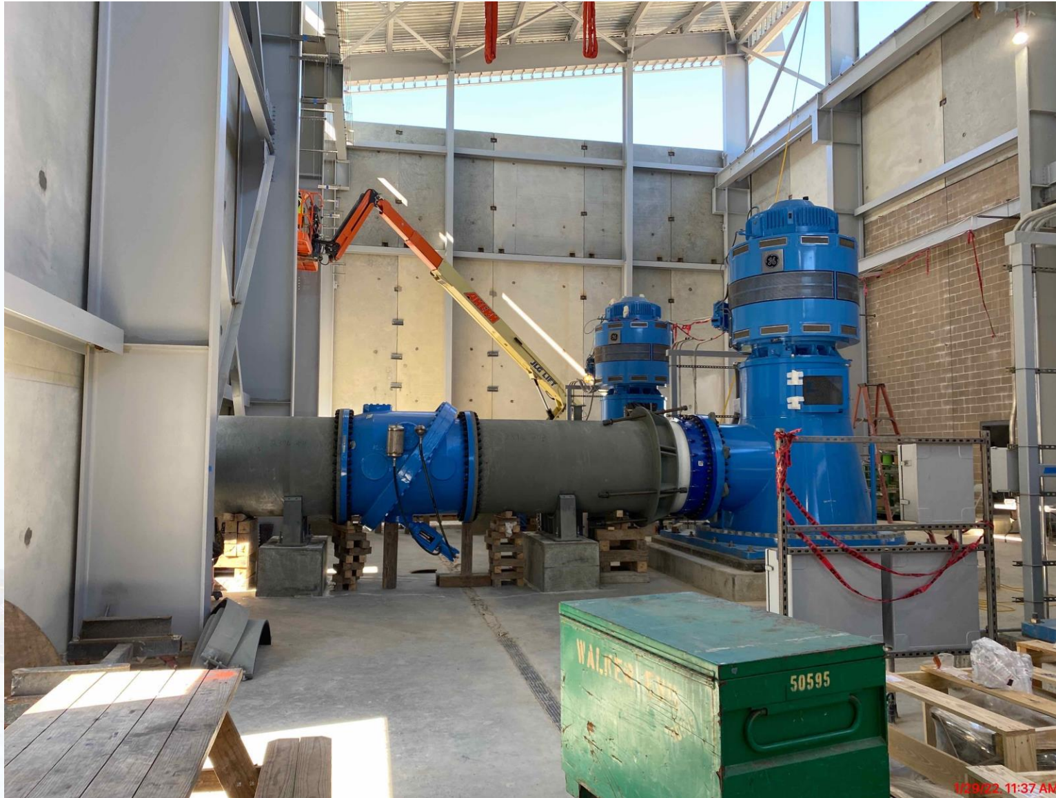
Continued 60" BWS connection and motor installation at Fac 401
