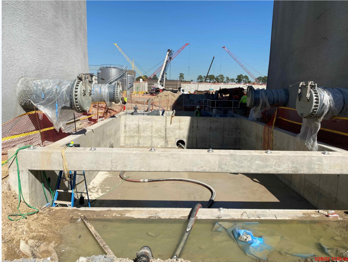
Resumed overflow box finishes (pipe, concrete invert, rails, and valves)
