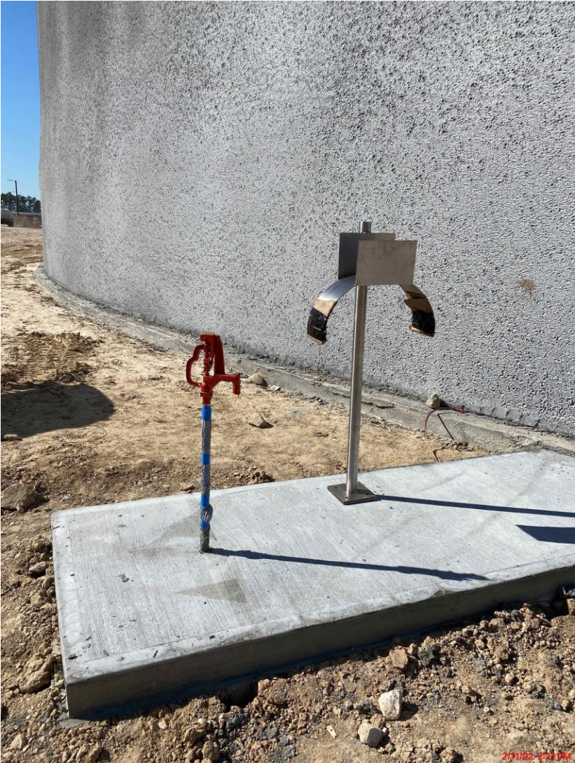
Commenced installation of hose racks and hose bibs
