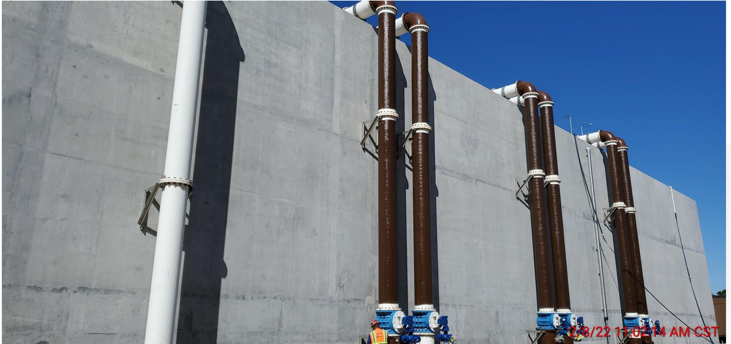
Continued process pipe installation at Fac 510.
