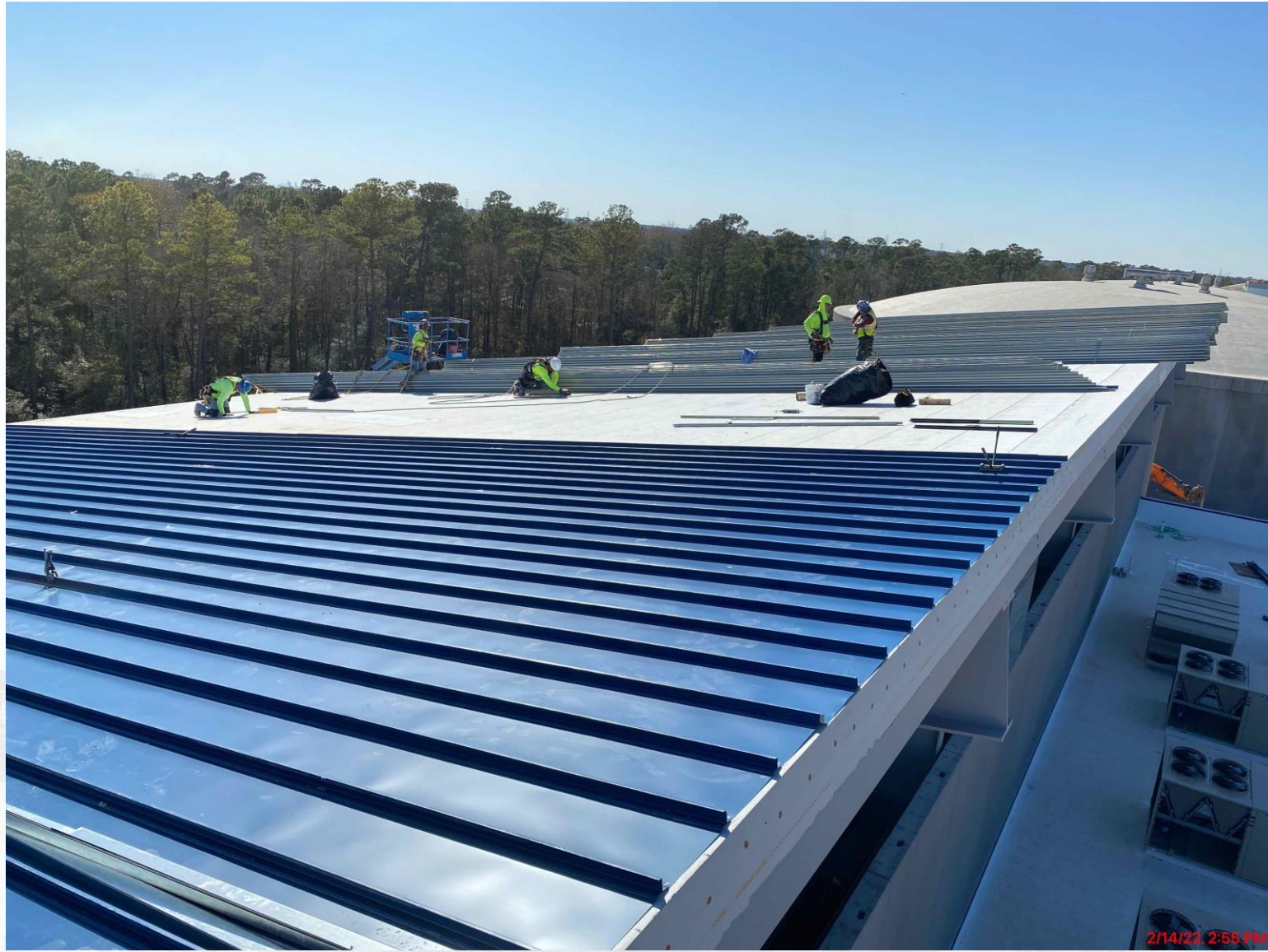
Continued roof installation at Fac 401
