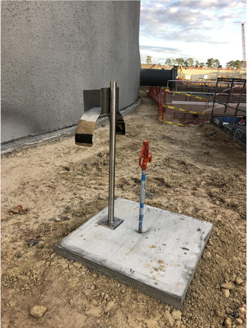
Commenced installation of hose racks and hose bibs
