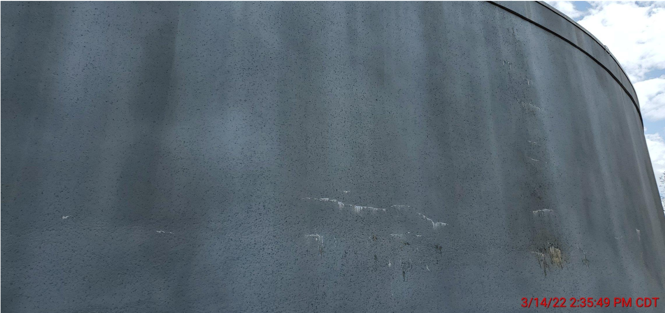
Completed tank wall repairs at GST 362
