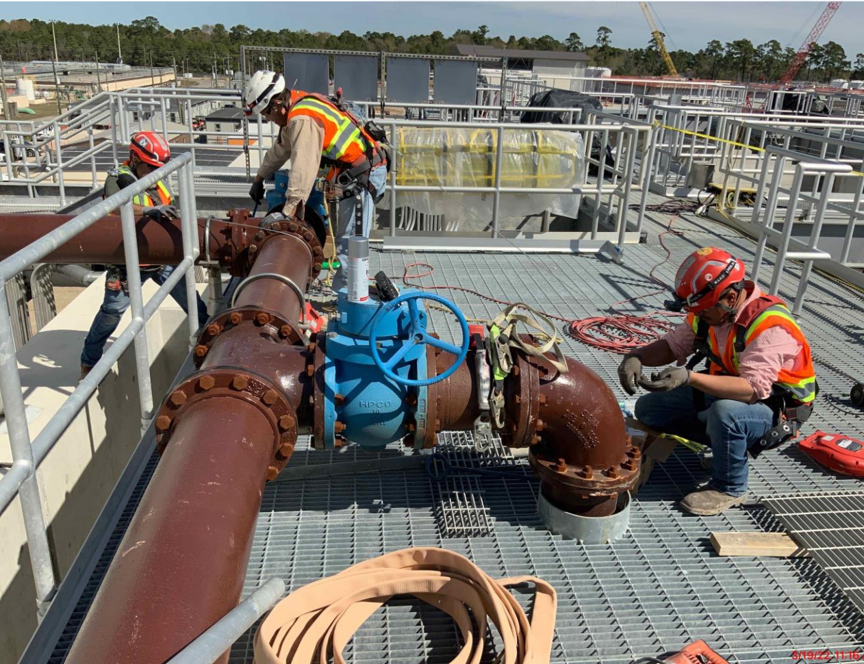
Continued process pipe installation at Fac 510.
