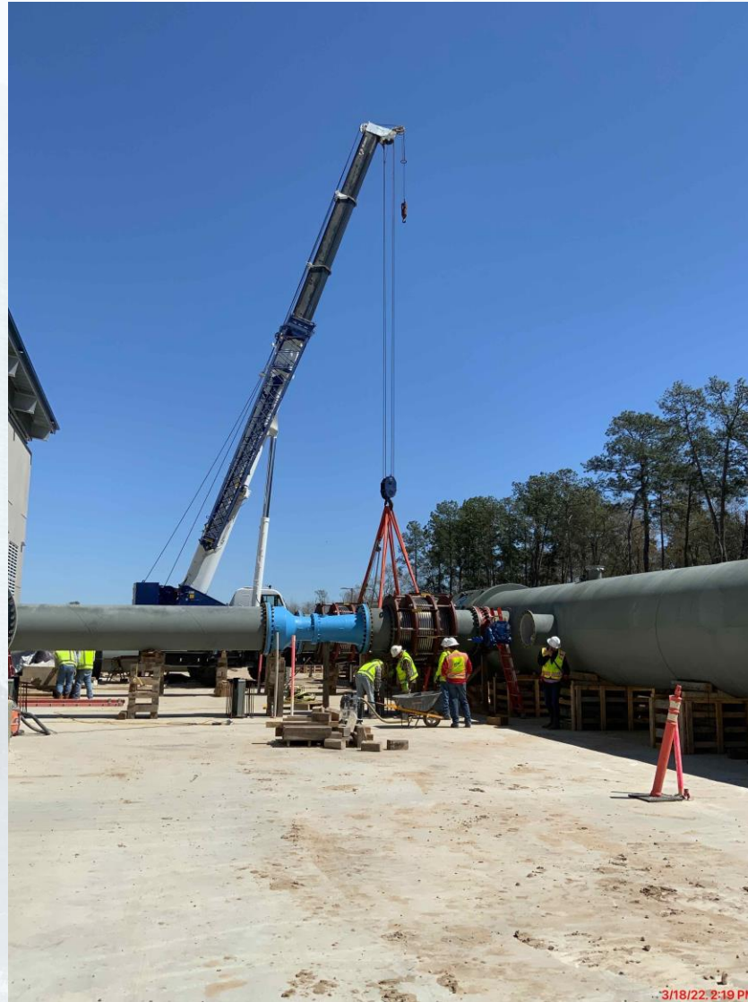
Continued installation of aboveground piping at Fac 401.
