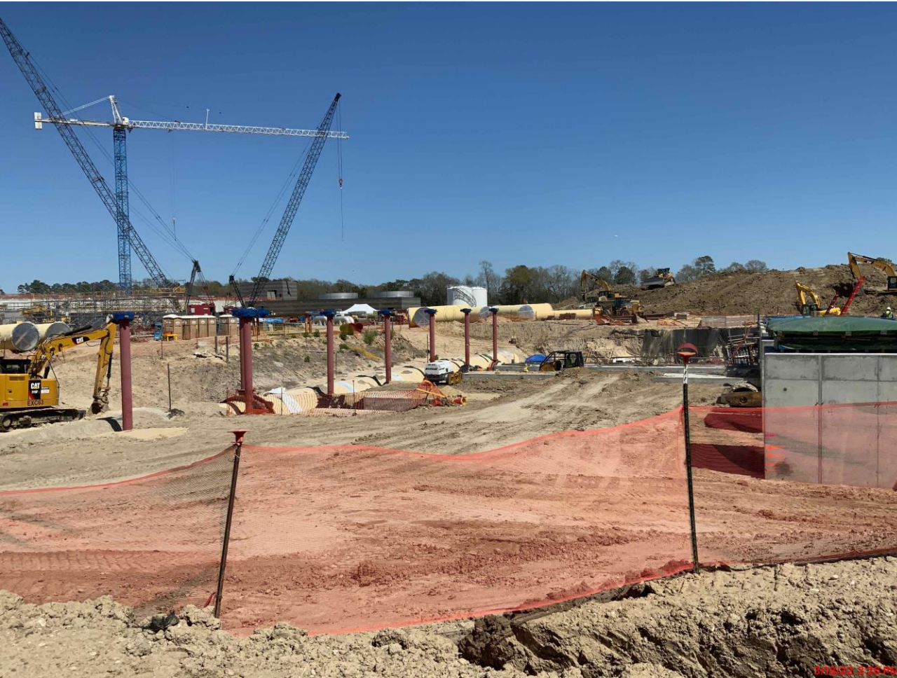
Continued backfilling and continued top of pump can encasement correction at Fac 402
