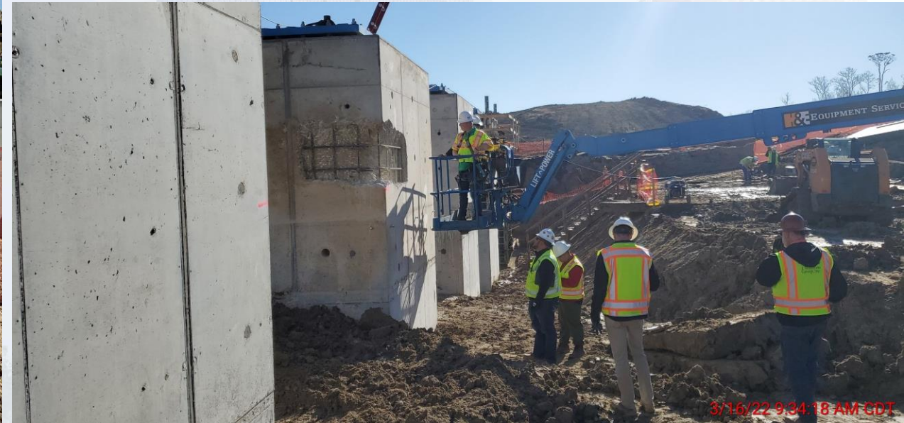
Continued backfilling and continued top of pump can encasement correction at Fac 402
