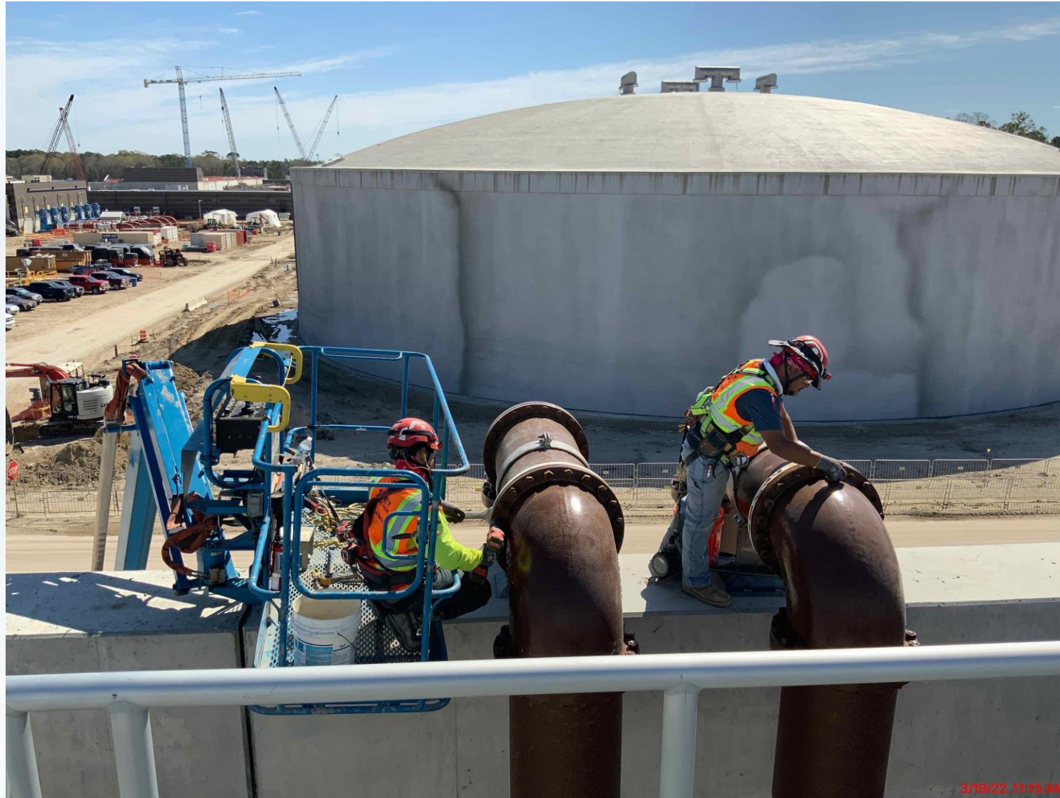
Continued process pipe installation at Fac 510.
