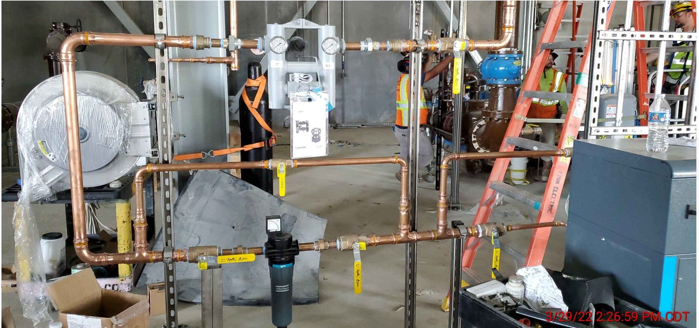
Continued installing plumbing, process pipe, and electrical conduit on levels 1, 2, and 3 at Fac 520
