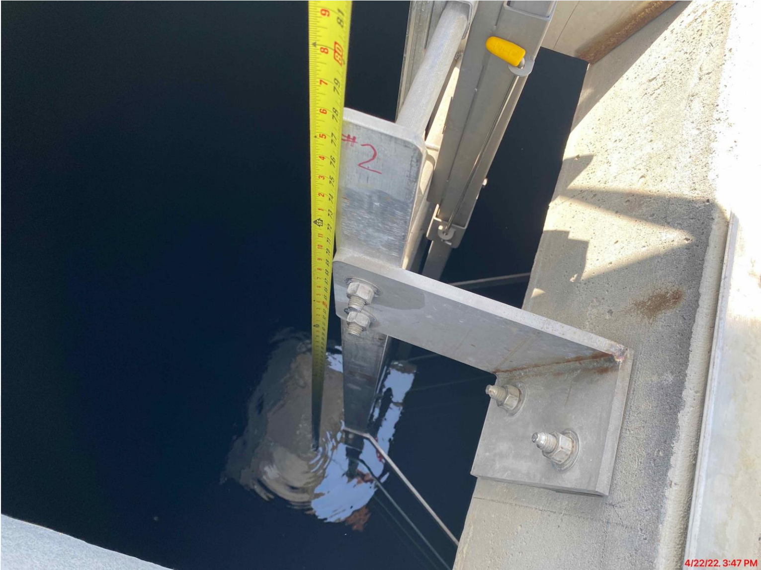
Watertightness testing at GST 362
