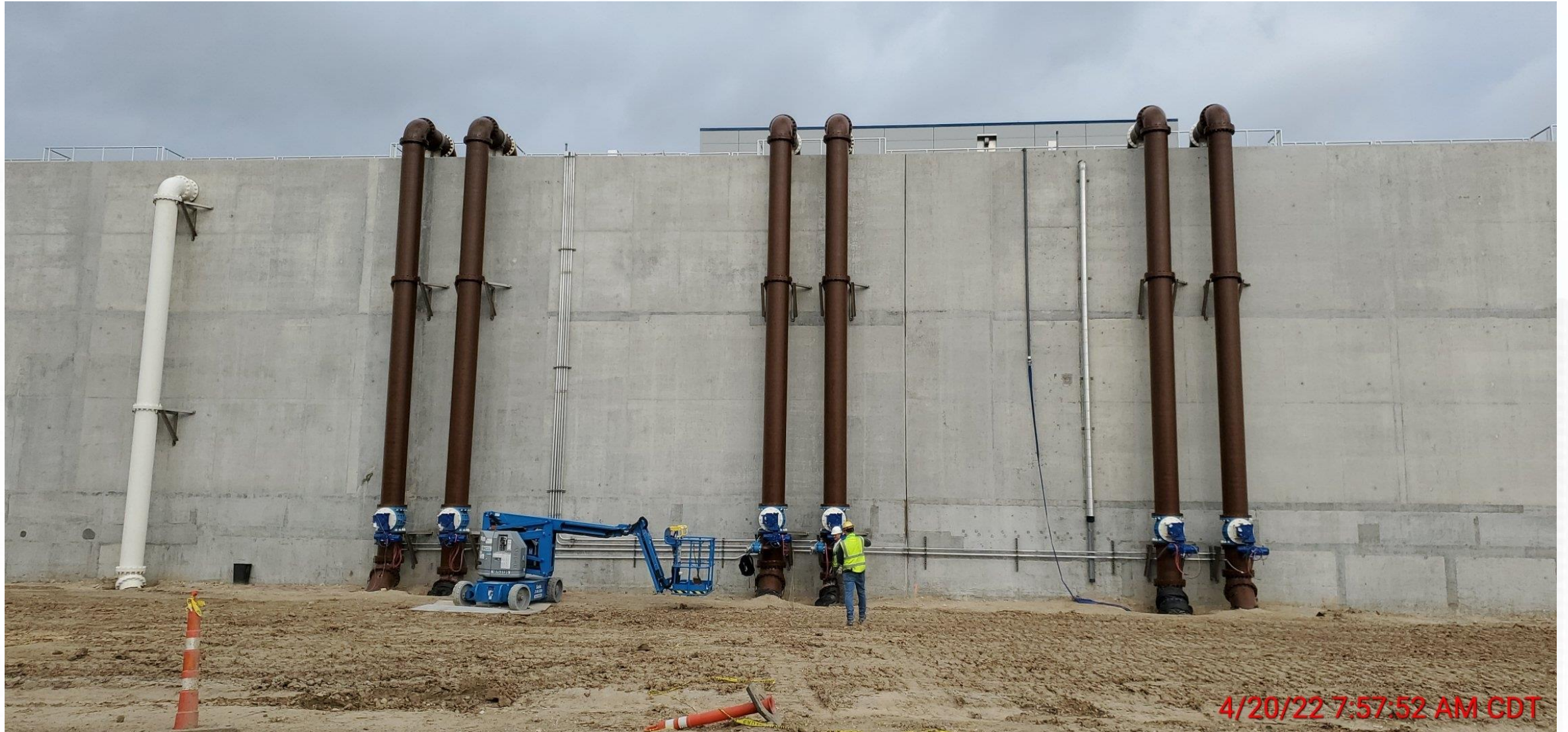
Continued process pipe installation at Fac 510.
