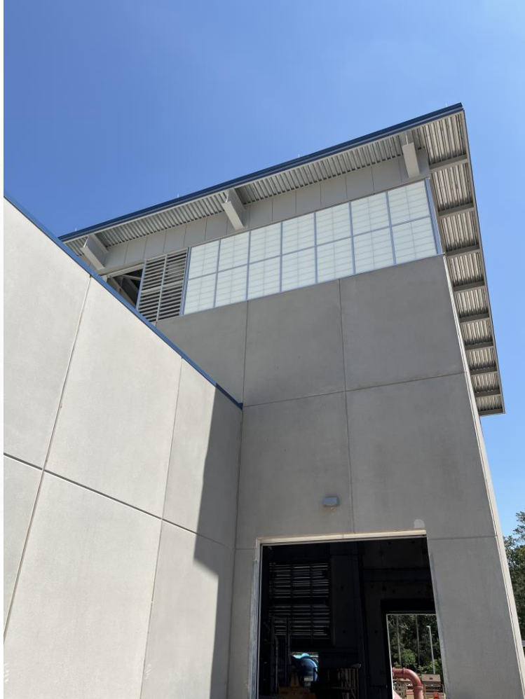
Installation of Translucent Panels
