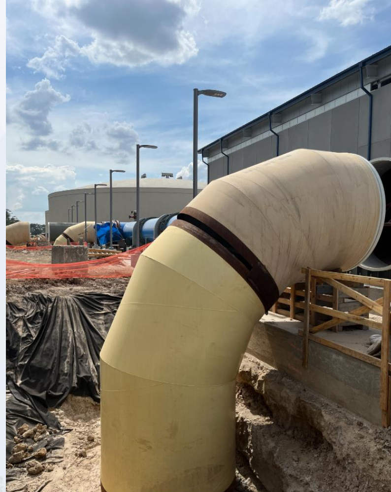
Continued installation of aboveground piping at Fac 401.
