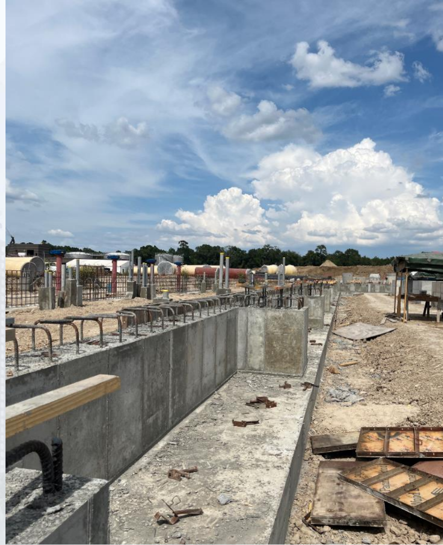
Pouring, rebar and form work Fac 402
