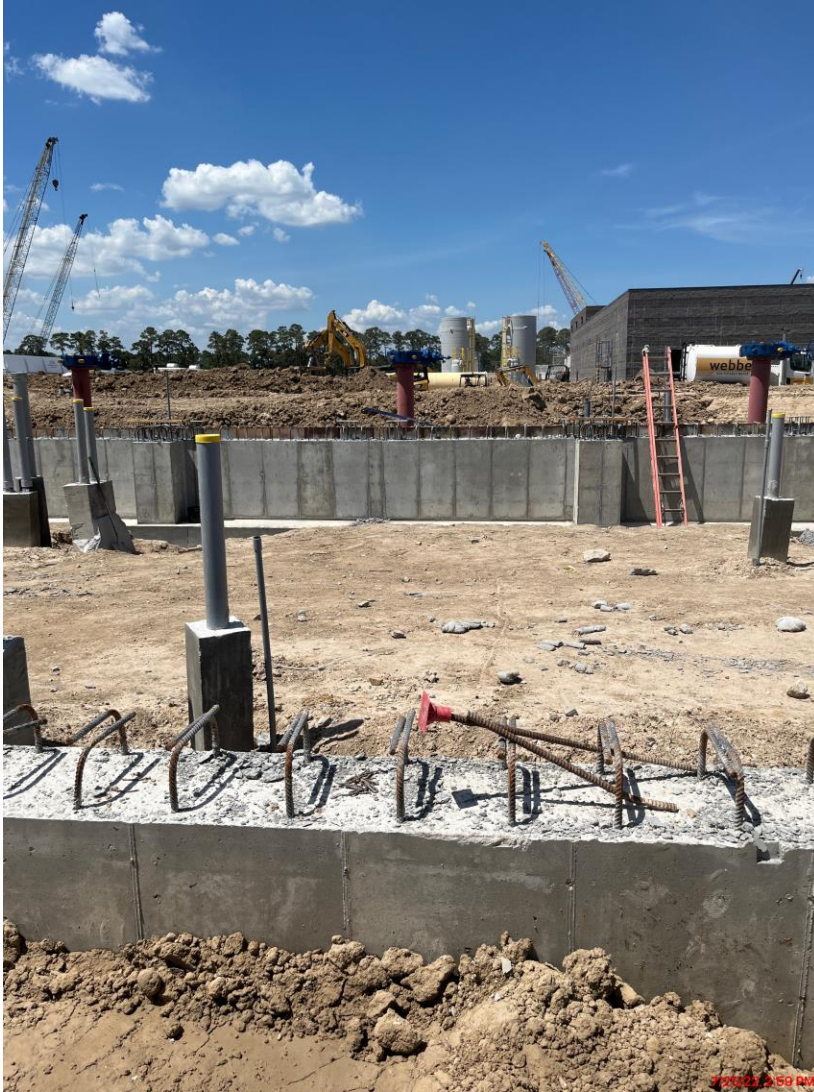
Pouring, rebar and form work on foundation
