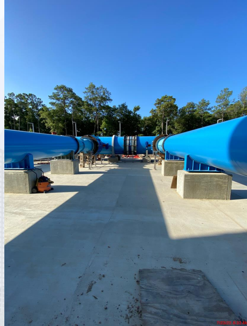
Installation of US Bellows and flow meters
