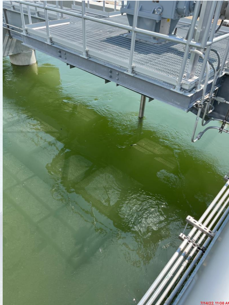
Mixer E&S testing at Fac 510.
