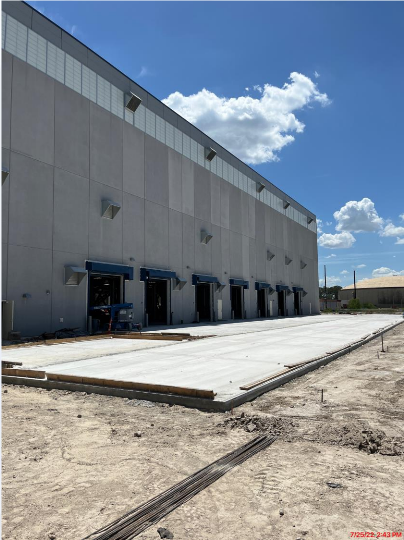
Truck Scales installation and conduit at Fac 520
