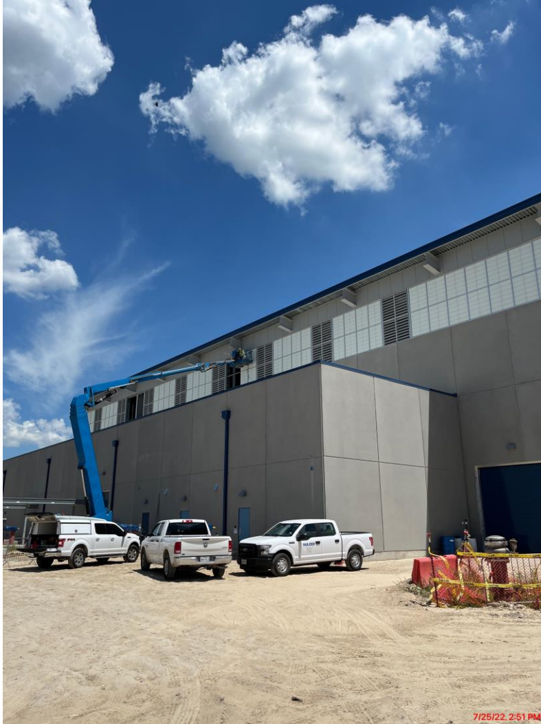
Continued Installation of Translucent Panels
