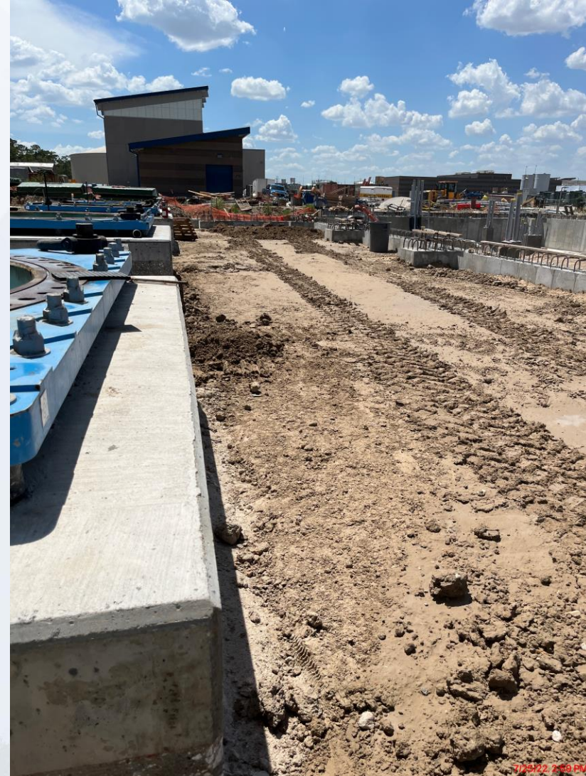
Backfilling at Fac 402
