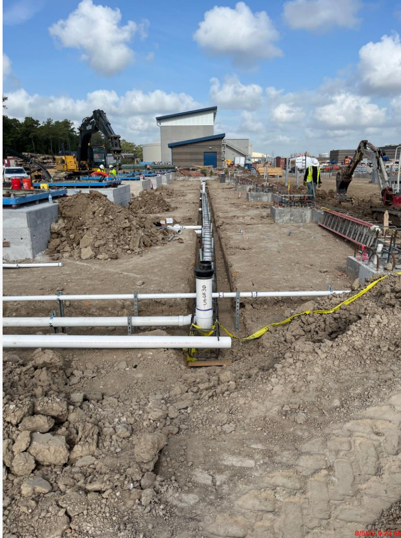
Pump room piping and embedded conduit installation
