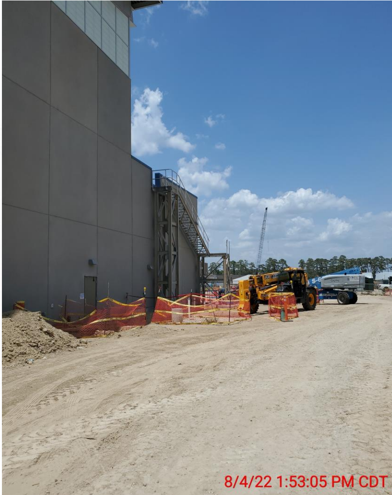
Installation of exterior stairs
