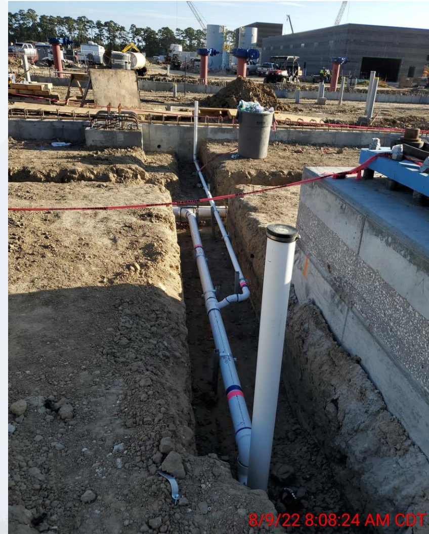
Pump room piping and embedded conduit installation
