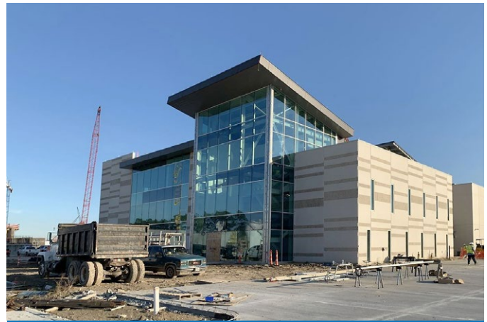
Completion of Curtain Wall Glazing
