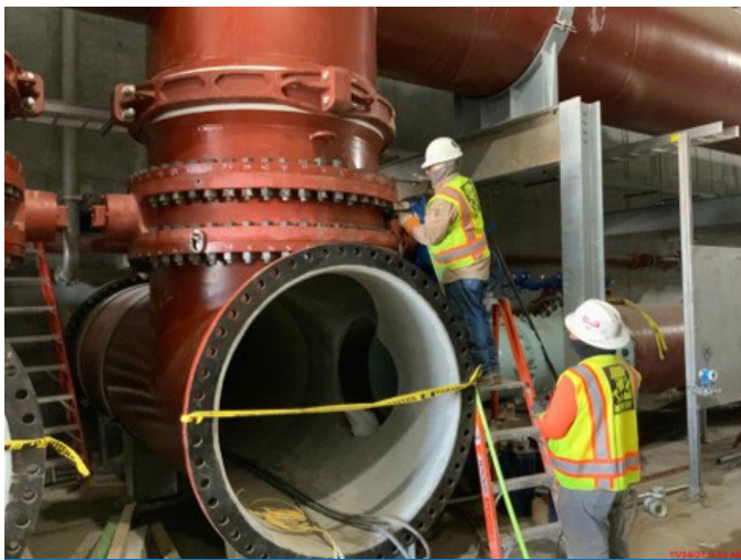
281 Filter Module – Finish Install Large Valves
