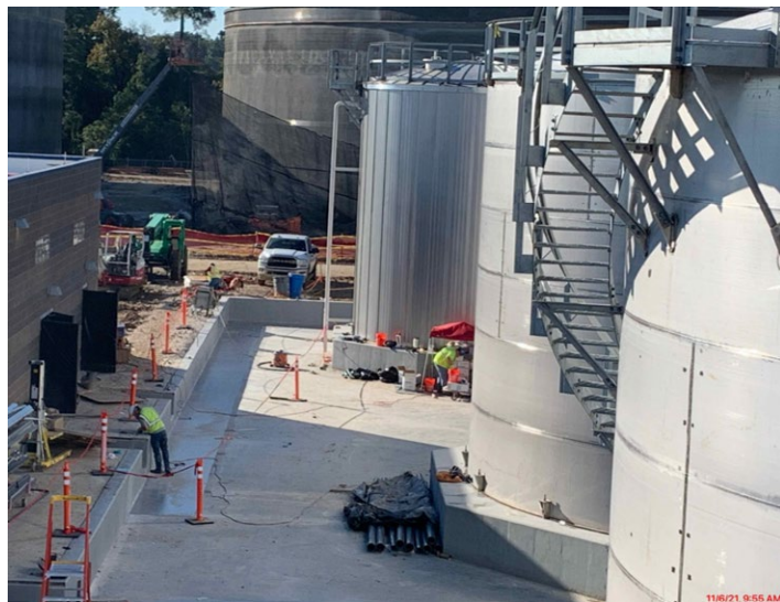
Facility 311 – CRC Surface Application
