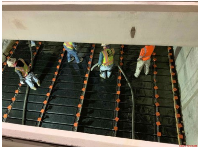
281-FILTER MODULE - Finish grouting Filter UD
