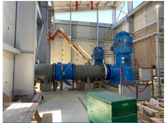
Motor Install HSPS 401
