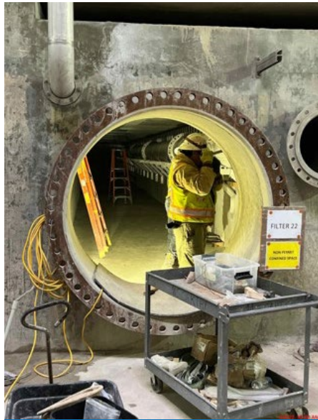
282-Filter Module 2 – Pipe installation
