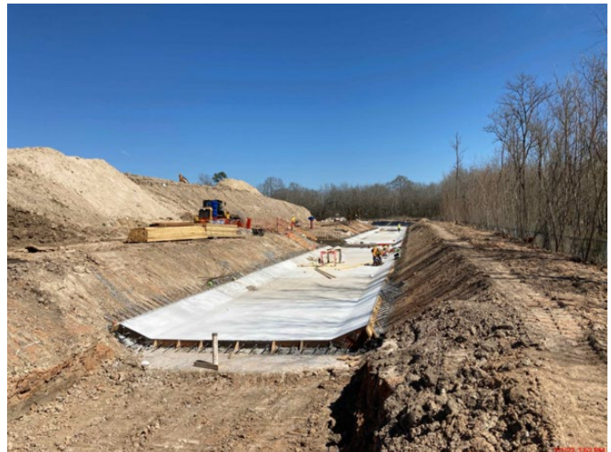
Overflow Channel Bottom Slab Installation
