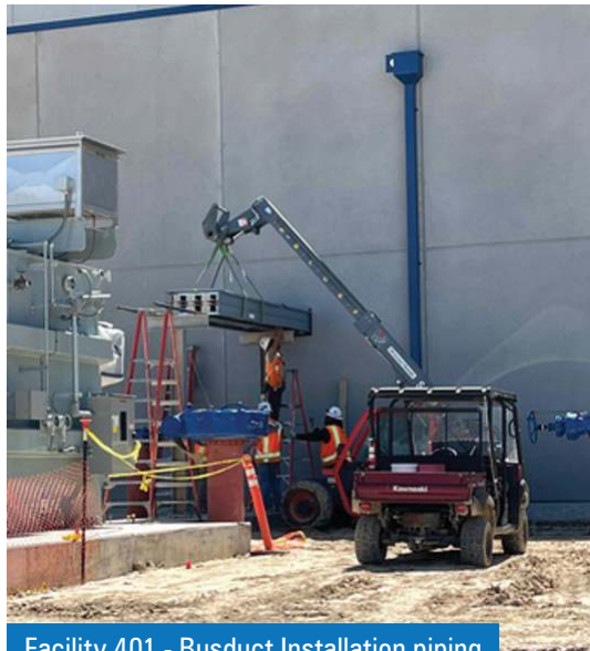
Facility 401 - Busduct Installation piping
