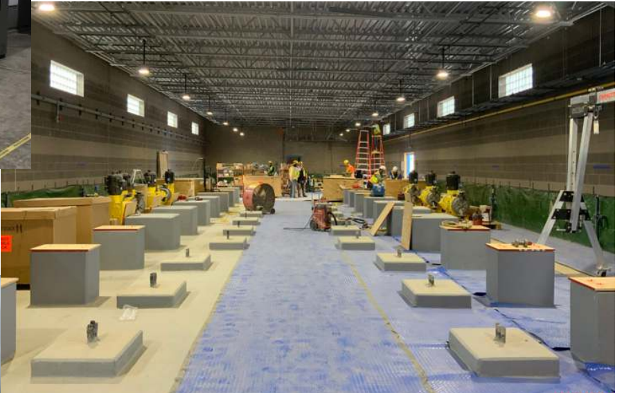
Facility 314 - Metering Pumps Installation
