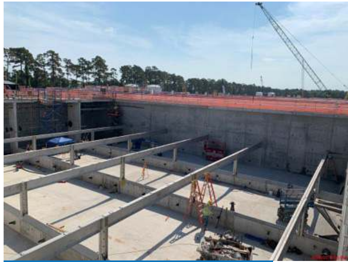
Facility 241 - Placement of Columns and Beams
