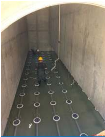
Facility 252 - Ozone Contactor 2: Diffuser Installation
