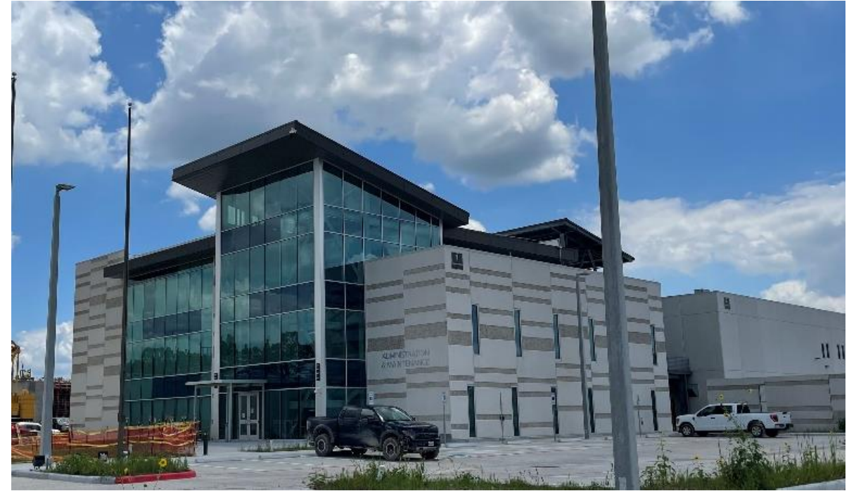
Administration Building nearly complete and move-in ready
